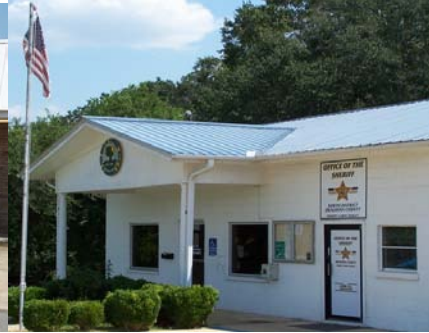
OCSO Laurel Hill Substation (adjacent to Laurel Hill City Hall)
