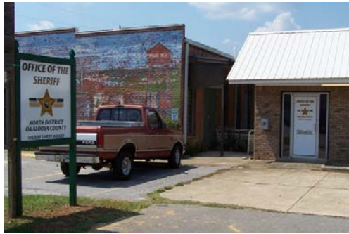
OCSO Baker Substation (across from Health Smart Pharmacy)
